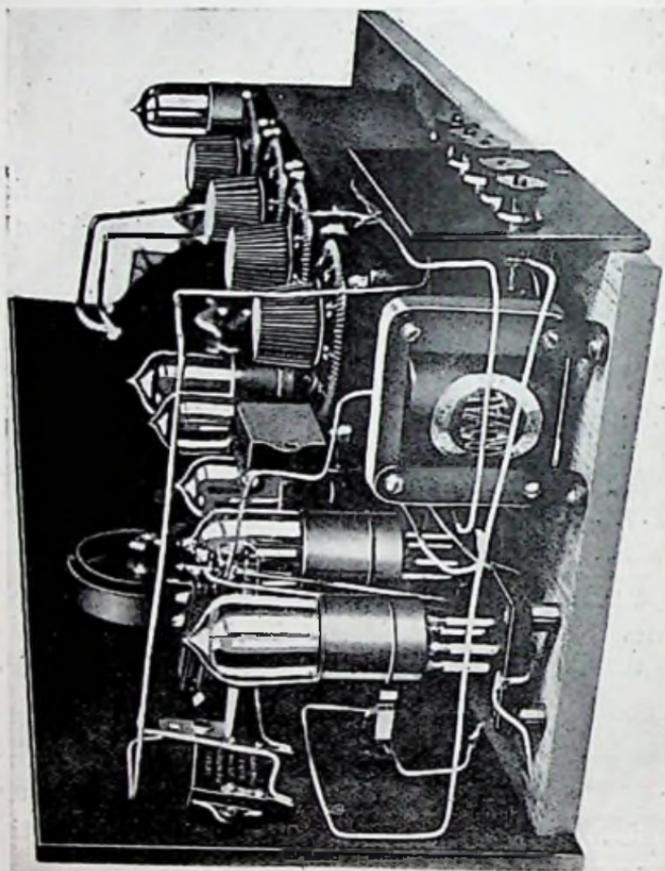
Fig. 24.—Back View of Tropadyne Receiver.
